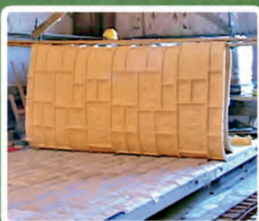
A power hoist is used to handle the 1,000 lb. (454 kg) liner.
