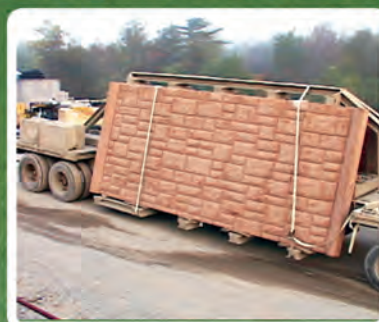
Completed sound panels are shipped to the job site.
