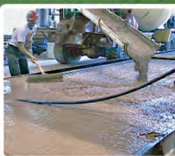
Concrete is poured into the mold. VytaFlex® offers excellent resistance to compressive loads.
