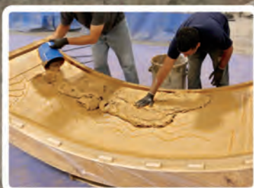
GFRG is applied into mold to create the decorative outdoor panel.
